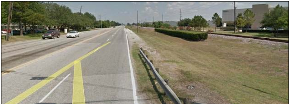
Figure 56 – Existing Configuration of Hempstead Road ROW at W. 34th Street/Kempwood Drive
